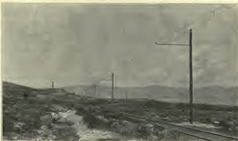
FIG. 528. OVERHEAD CONTACT SYSTEMS. Single Catenary 2,400-Volt Direct Current Main Line Construction, Butte, Anaconda & Pacific Railway.
